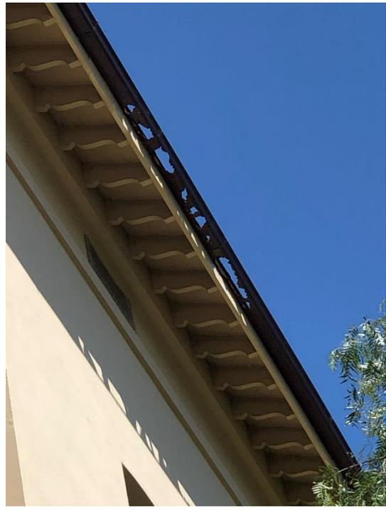
Figure 4 - Severely corroded gutter to North side of unit 135
