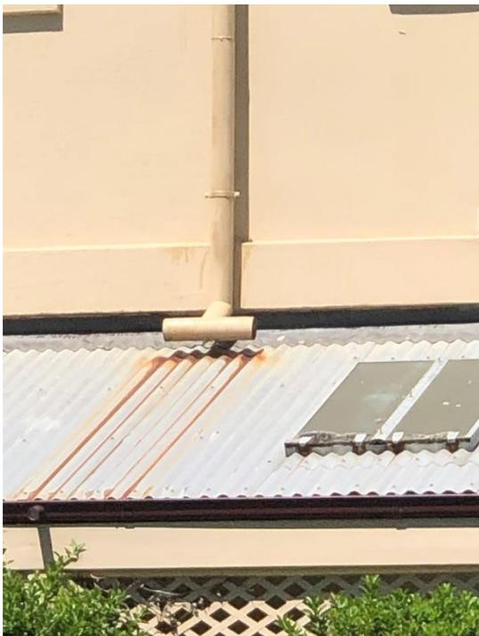
Figure 2 – Typical Staining to verandah roofs found at the base of downpipe spreaders from roofs above.
