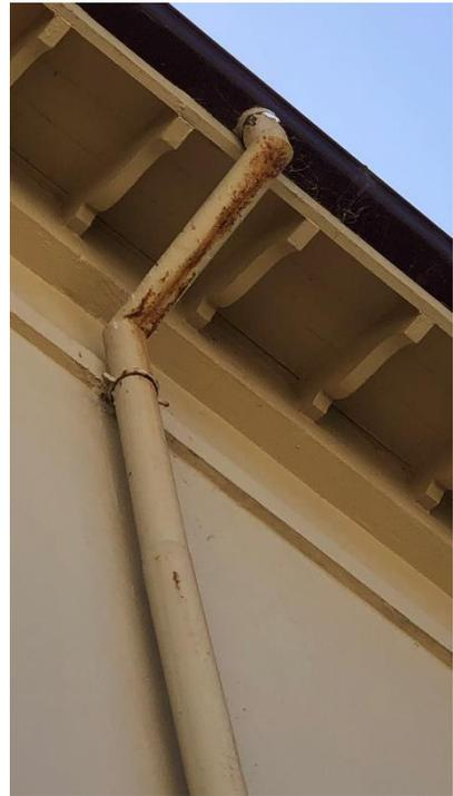
Figure 5 – Downpipe located on east side of unit 135 showing heavy corrosion and detachment from gutter.
