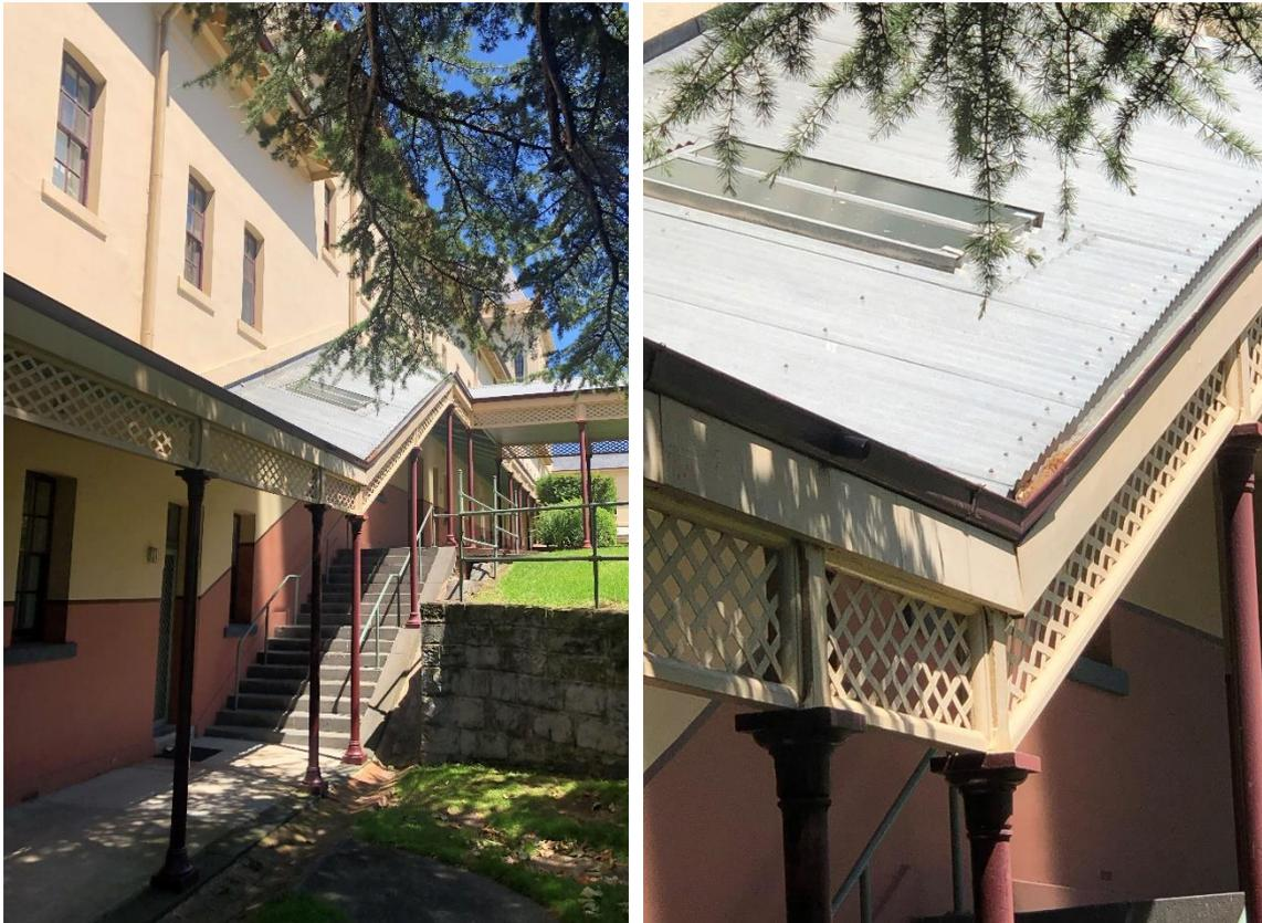
Figure 6 - Build-up of leaves / debris in verandah eave gutter outside unit 130 note proximity to tree.
